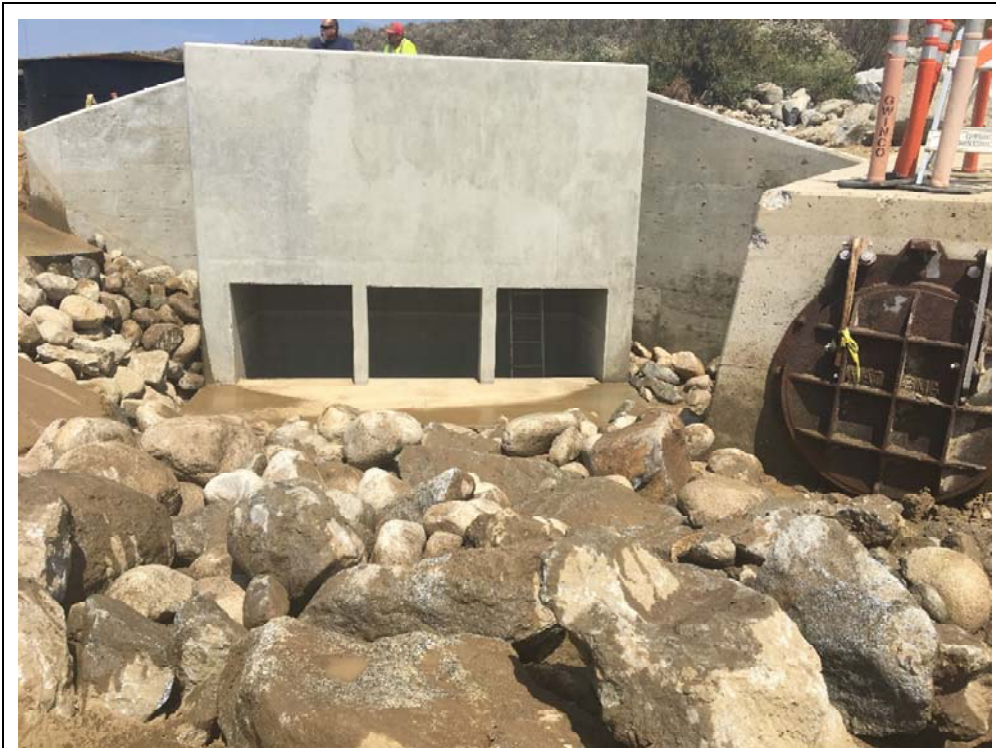
Installed new stormwater inlet structure
