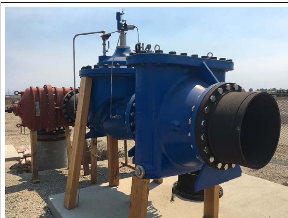
Installation of new strainer and control valve at the Recycled Turnout
