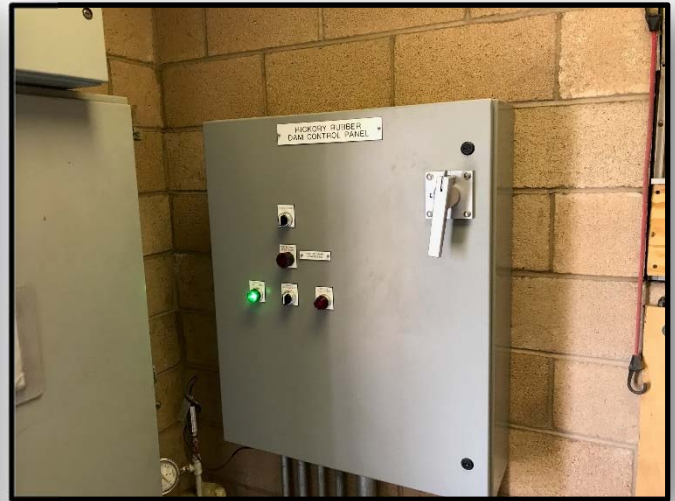
Rubber Dam control panel
